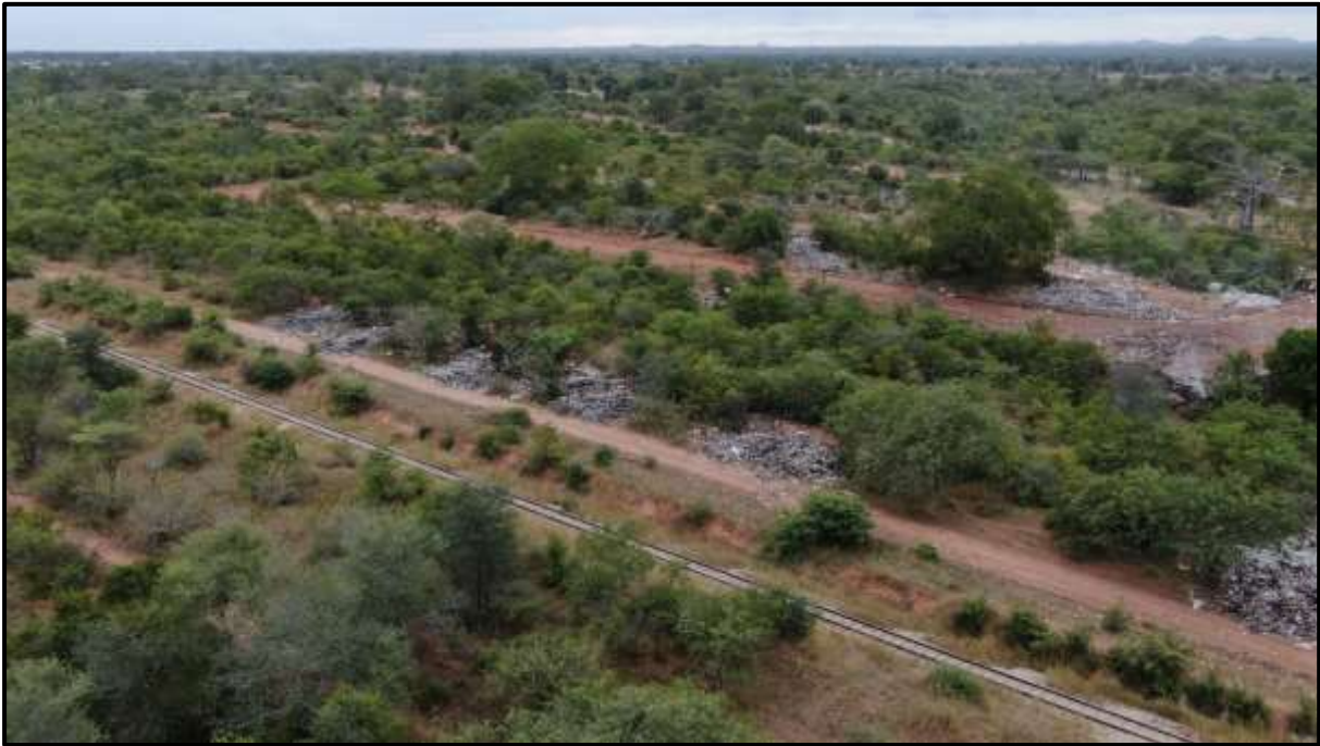
Plate 23: Dumping of solid waste along railway line ( Survey, 2024 ).
