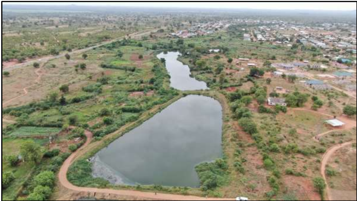
Plate 21a: Ariel view of Chiredzi Sewer Ponds ( Survey, 2024 ).
