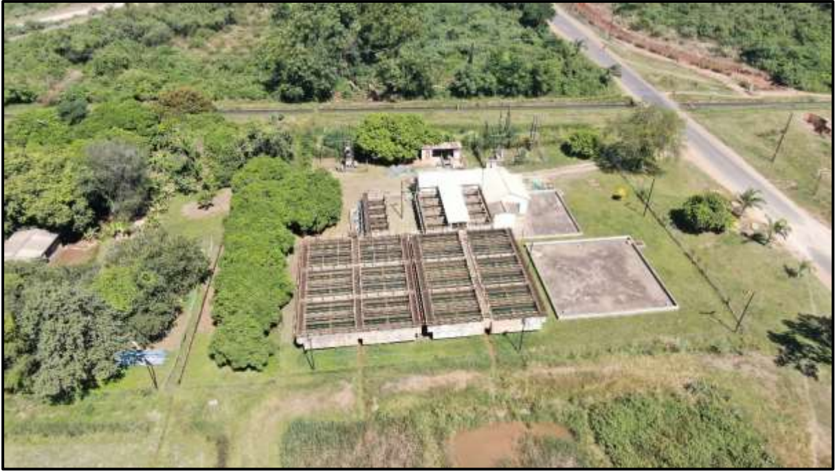
Plate 20: Water works ( Survey, 2024 ).
