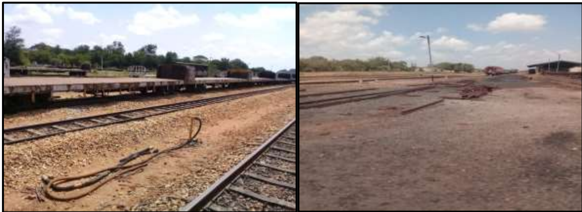
Plate 25: Railway line in Chiredzi ( Survey, 2024 ).
