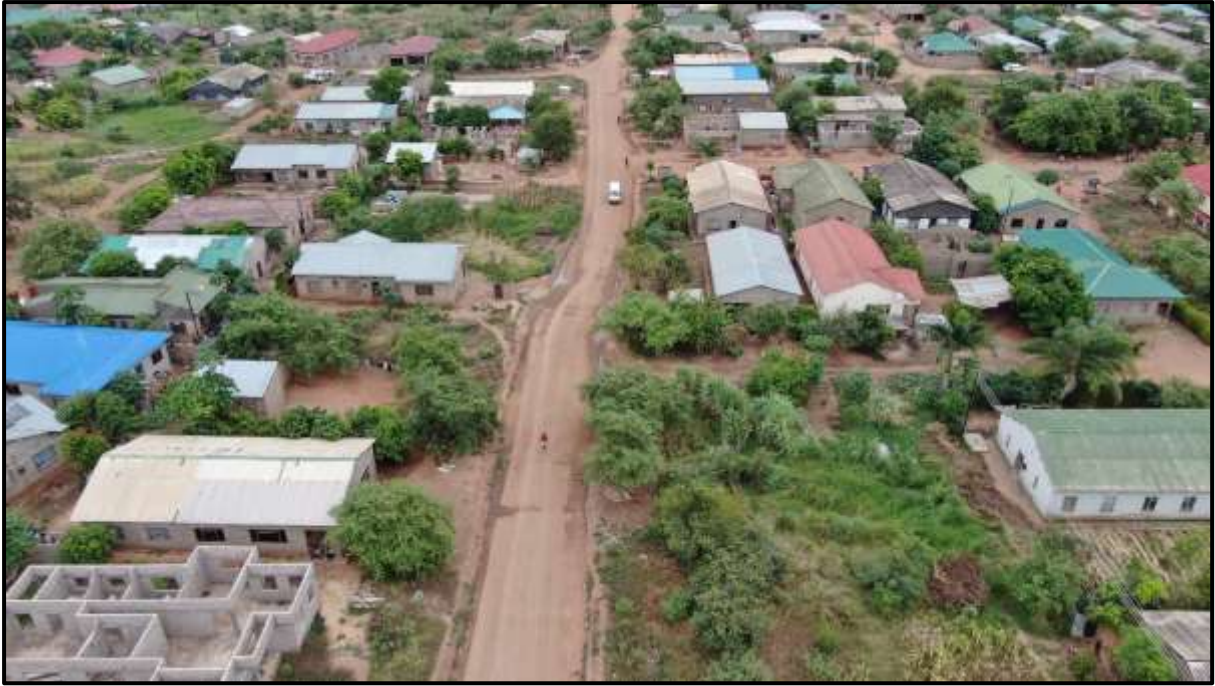
Plate 12: Unsurfaced Road in residential area in New Makondo ( Survey, 2024 ).
