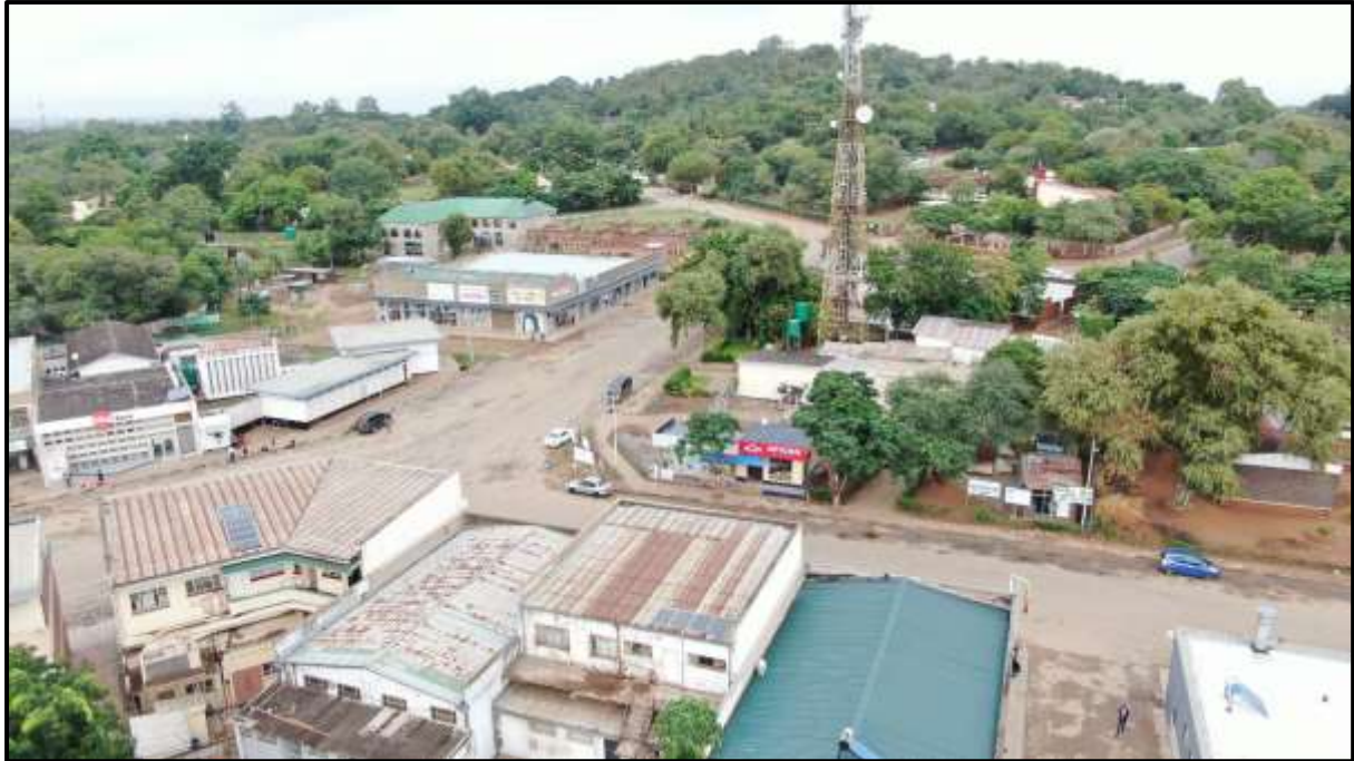
Plate 24: Telecommunication booster in the CBD ( Survey, 2024 ).
